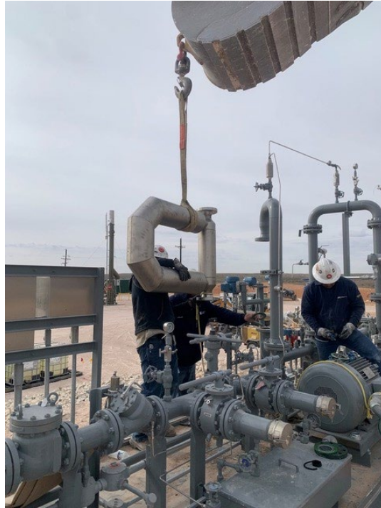
Figure 2. Coriolis being removed from a pipeline.
