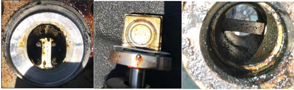
**Figure 3: e9 Pro Performance treated 2" Vortex meter with minimal deposition after 80 days of operations.**
